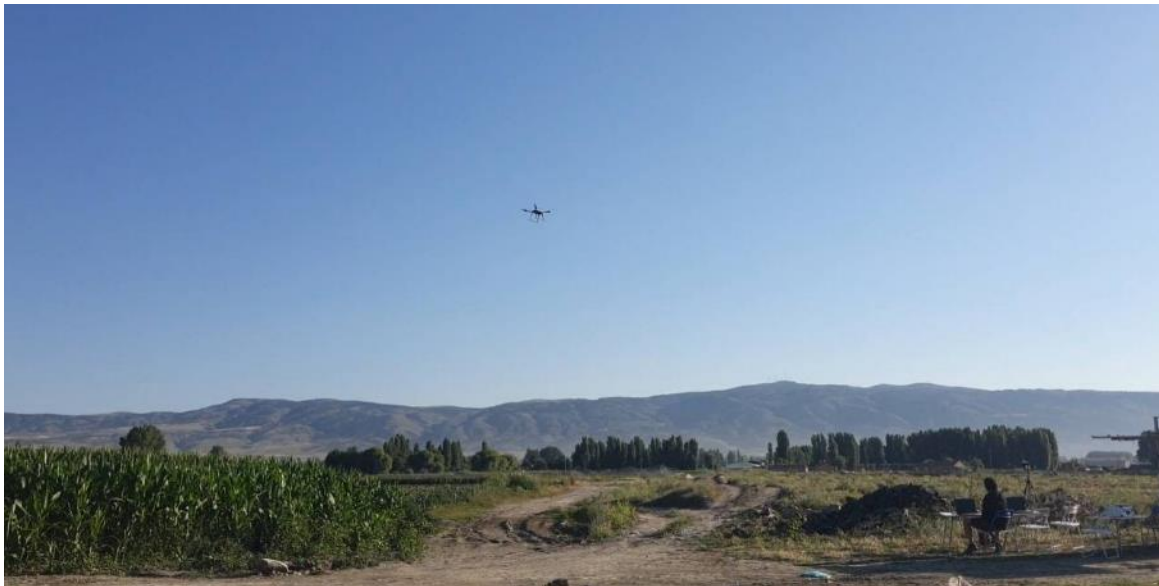
Figure 27. Pre-execution drone flights and ground control station on site
