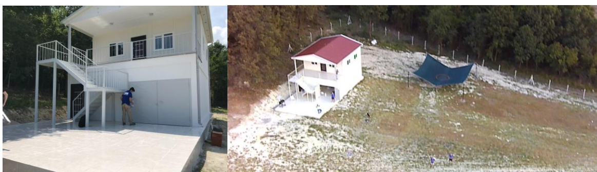
Figure 10. Ground and aerial photos of ITUARC Orencik UAV Test Field
